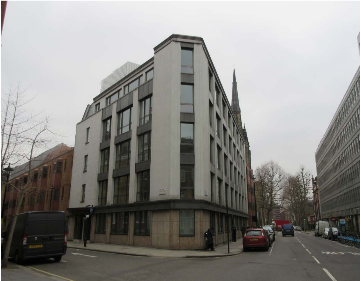
Front view of 33 Greycoat Street prior to works to convert to residential commencing.
